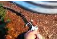
Using air to drain pipes
