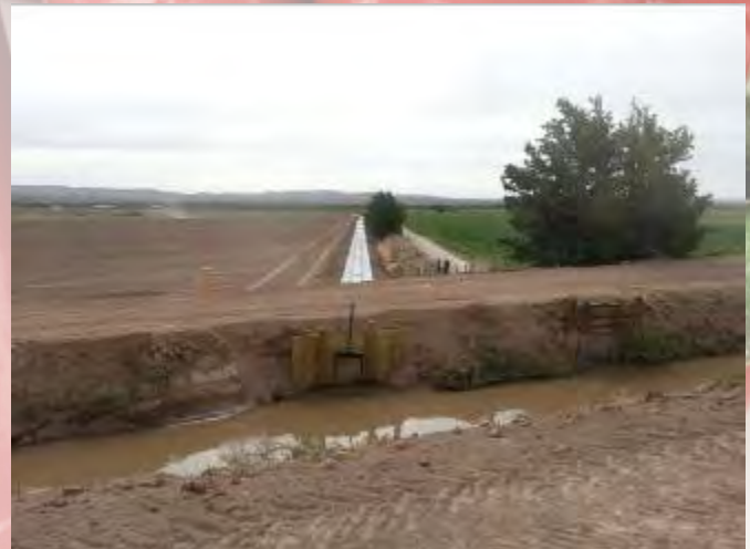
Newly replaced turnout
