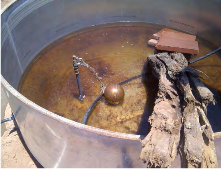
Stock tank with wildlife escape ramp. Water is pumped up to fill stock tank, then feeds drip irrigation tubing to water native shrub and tree plantings.
