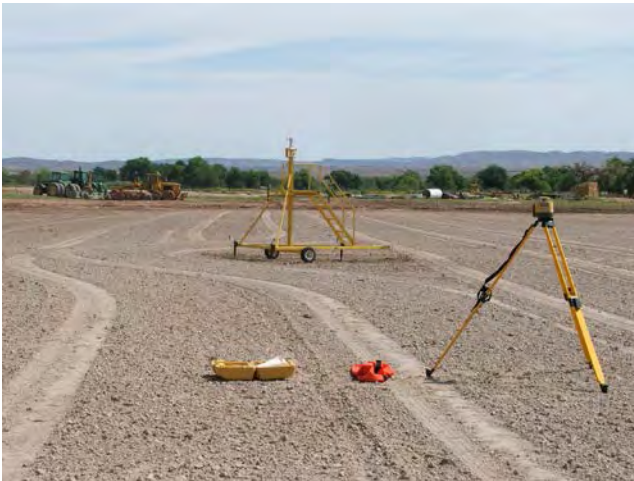
Laser leveling and survey equipment
